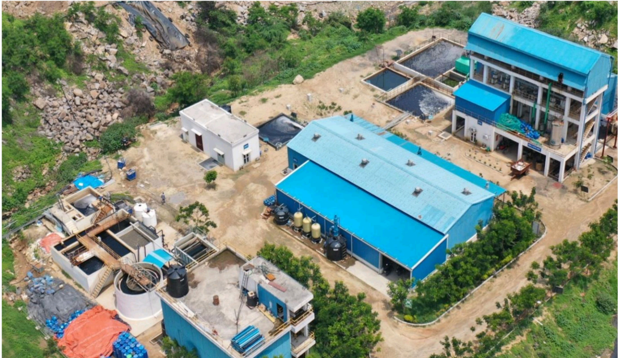
Waste Water Treatment plant (leachate treatment)
