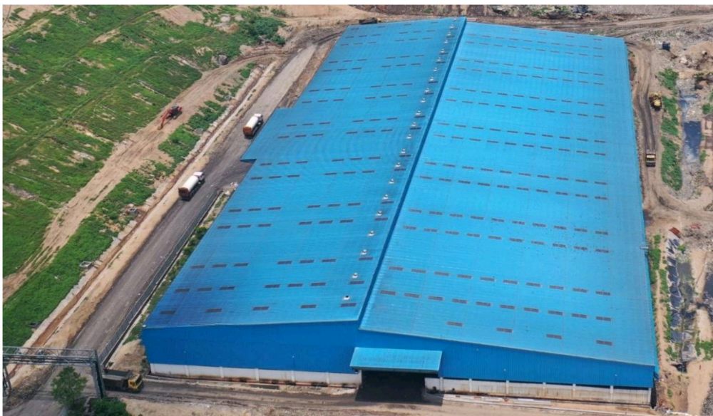
Closed Tipping floor & Pre-sorting facility
