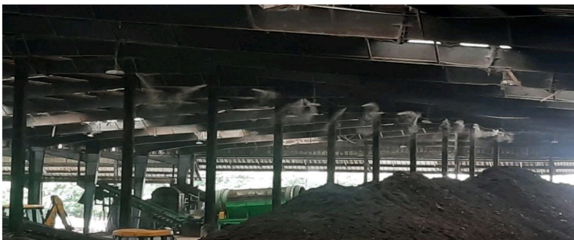
Spraying through fixed misting lines near presorting, composing areas, leachate storage etc
